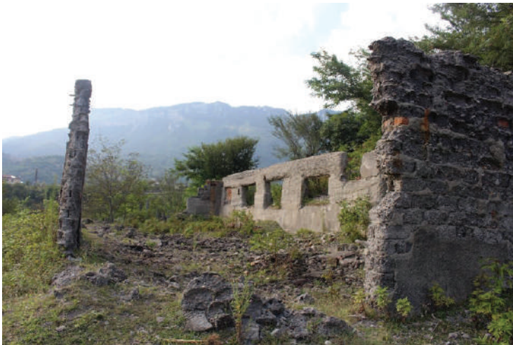
61. Barrack remains at the site of Tkibuli mine camp (Georgia)
